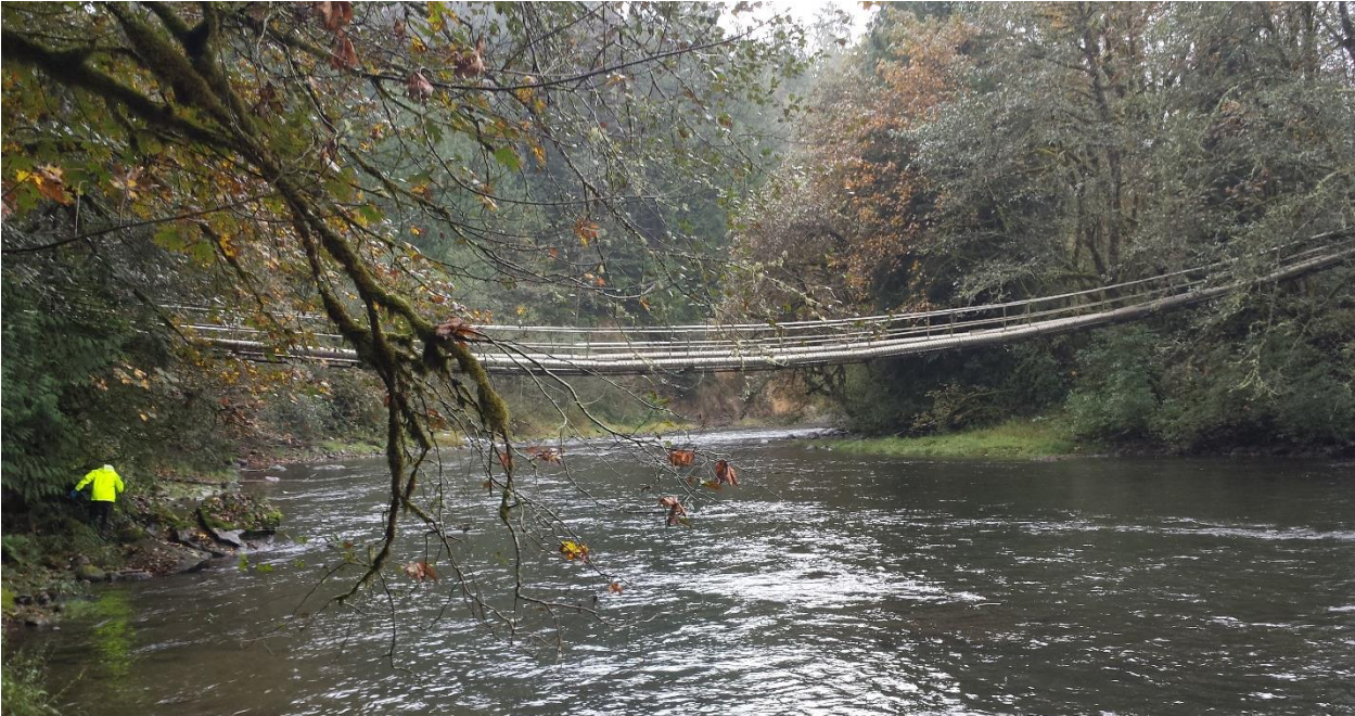
Green River Pipe Bridge
