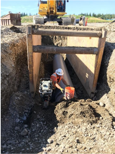
Large Diameter Water Main Installation
