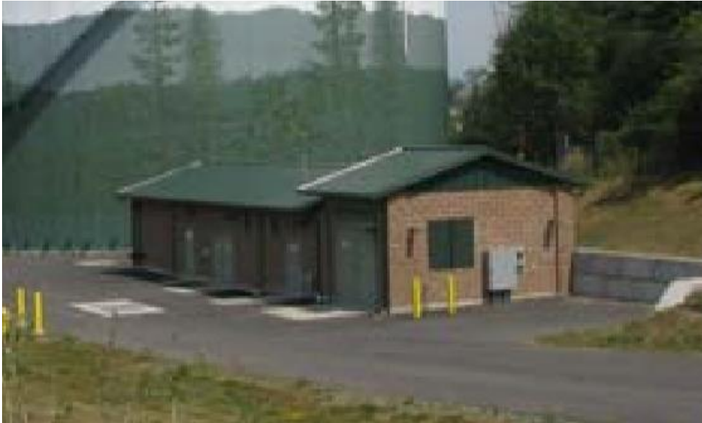
4.3 MG Reservoir Pump Station and Treatment Building
