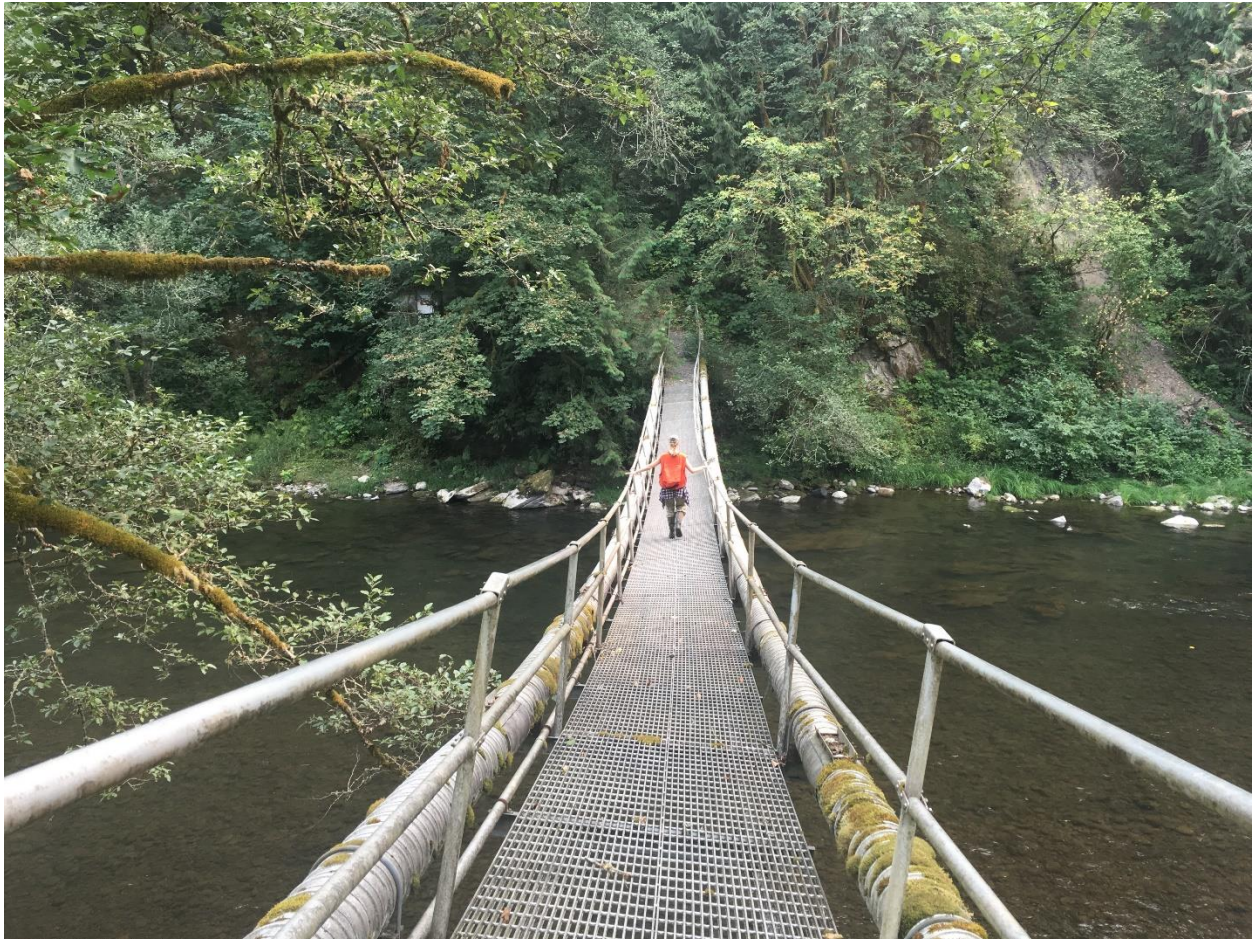
Green River Pipe Bridge
